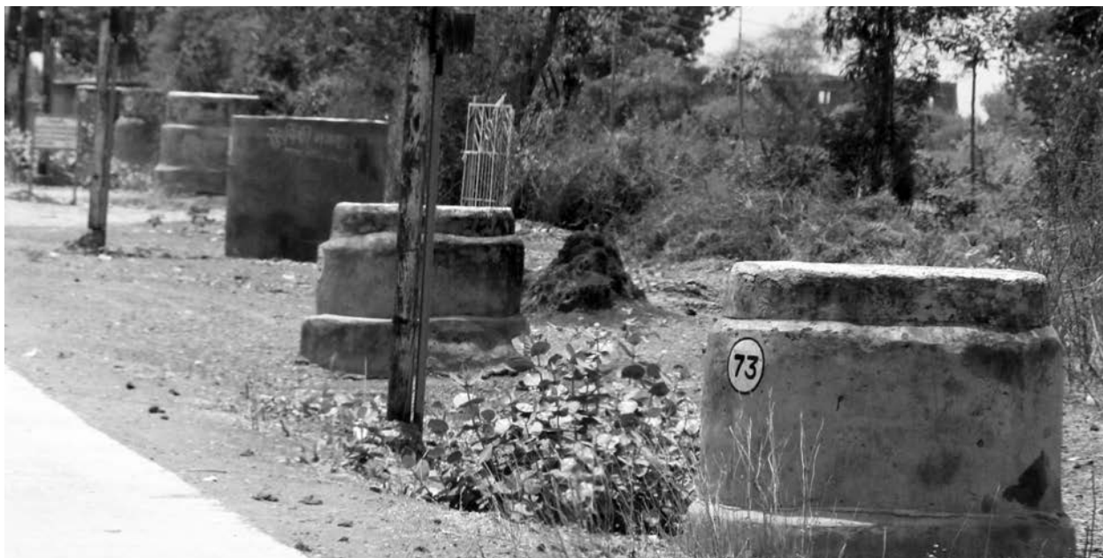
Air shaft on the surface of qanats also used as wells, Burhanpur 2
