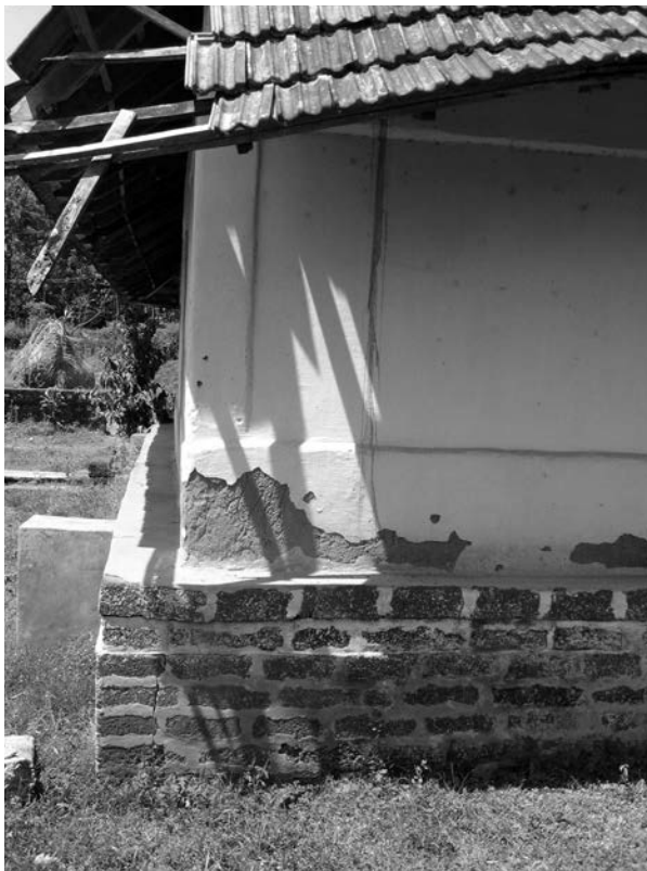
Detail of mud wall, lime plaster and laterite plinth
