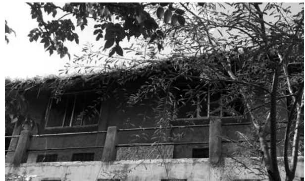
Sliding glass windows being fit to protect from extreme winds and simultaneously maintain the view from the house
