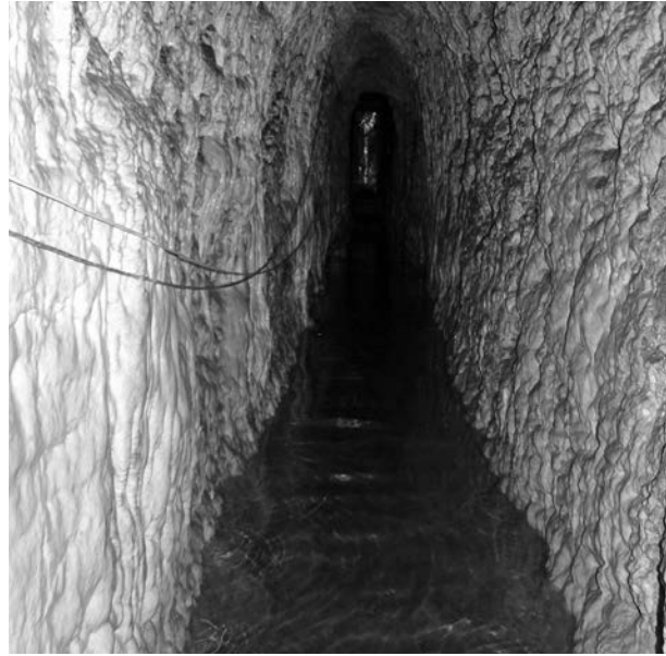
The subterranean water tunnel carrying water from the Khooni Bhandara to the town areas 9
