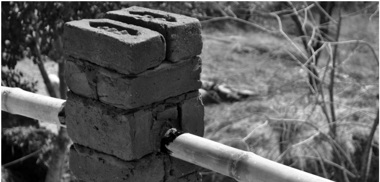
Bamboo embedded into pillars
