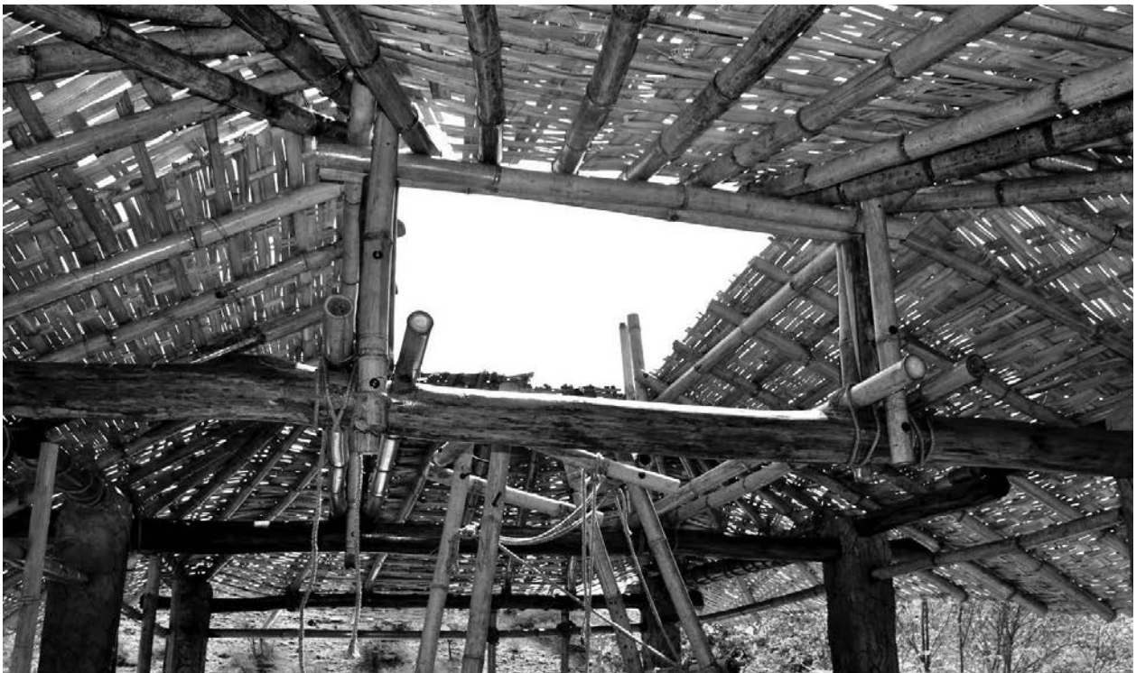
Interior framework of ceiling
