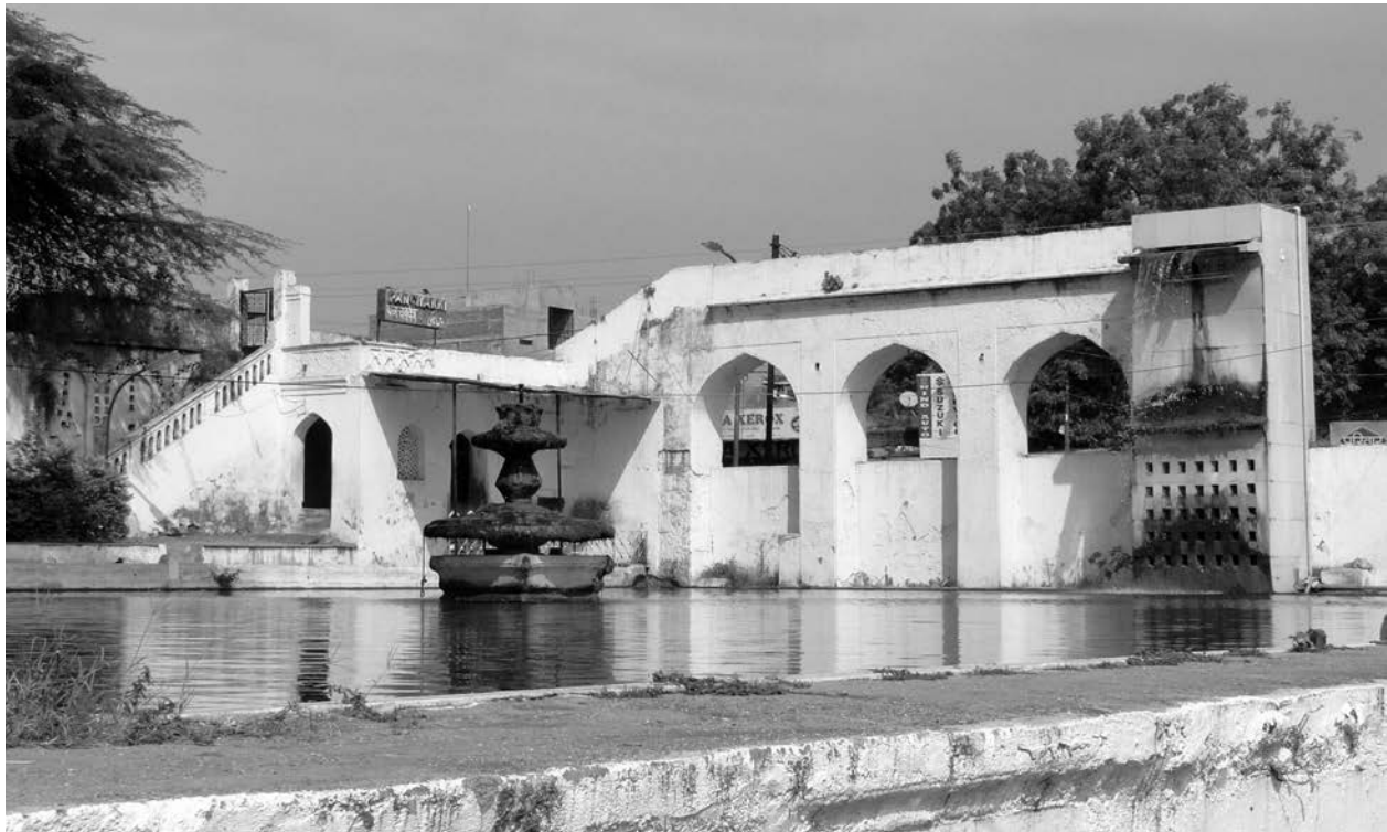
Nahar-e-Panchakki which brings water to this site through the wall in front. In the past a flour mill was run using incoming waters
