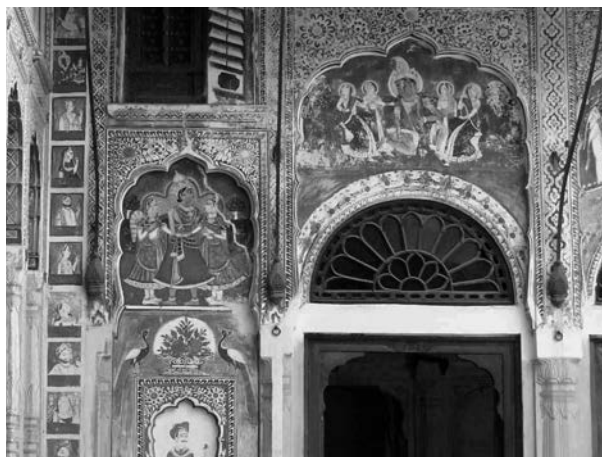
Coloured glass used in semi circular opening
