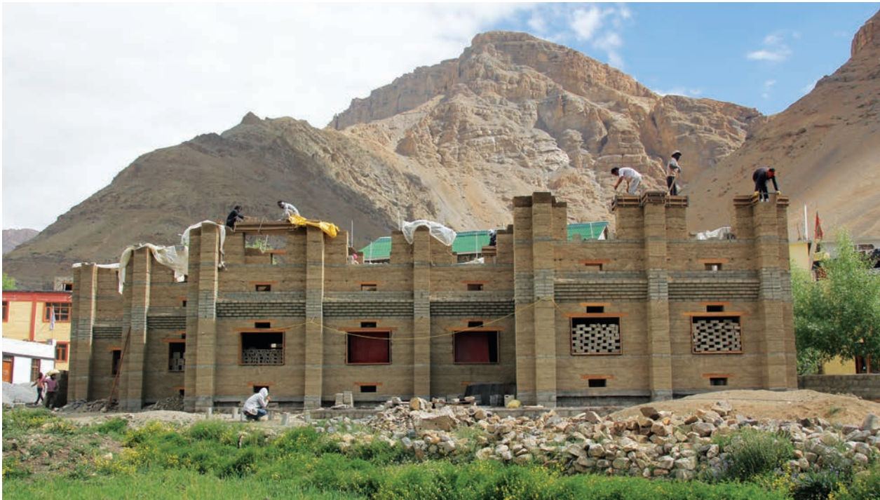
The construction of the Kaza Community Centre nearing completion
