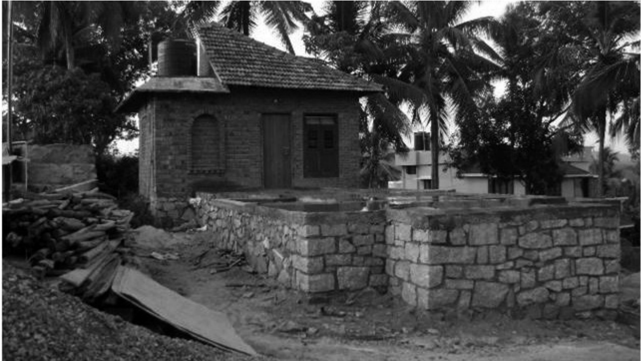
Initial portion and foundation in mud mortar
