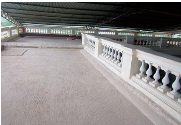
Finished Madras terrace from above. Source: RGRA project in Aneondi, Karnataka
