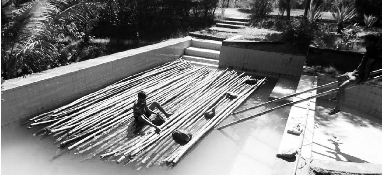
Bamboo treatment by soaking it in lime and salt water
