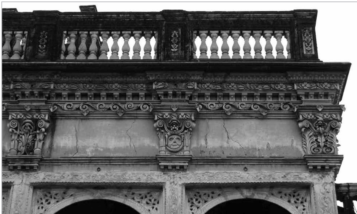
Stucco plaster on facade
