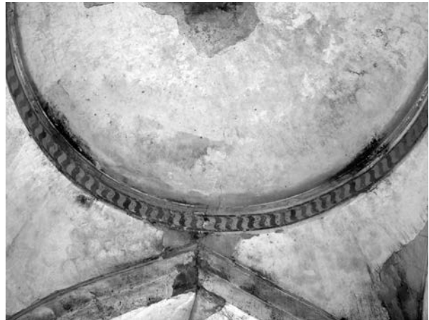
Band of tiles on ground floor domical ceiling seen in Jahaaz Mahal in Mandu
