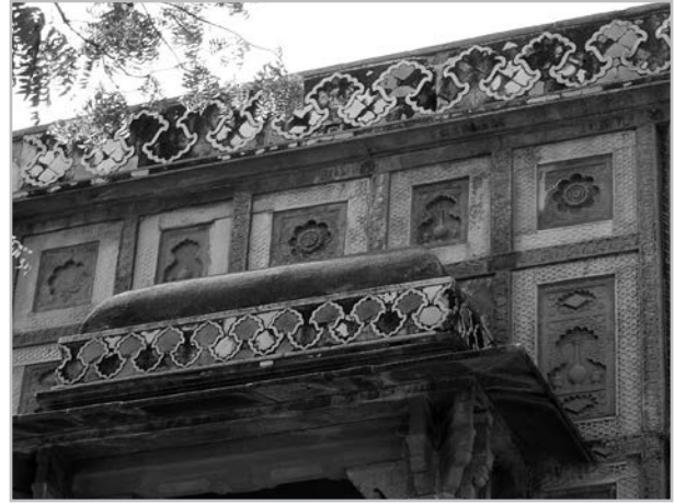
Tilework on parapet and roof of balcony, Kanch Mahal, Agra
