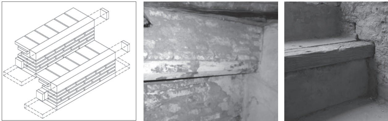
Construction detail of staircase using wooden joist and traditional masonry in nanakshahi bricks and lime
