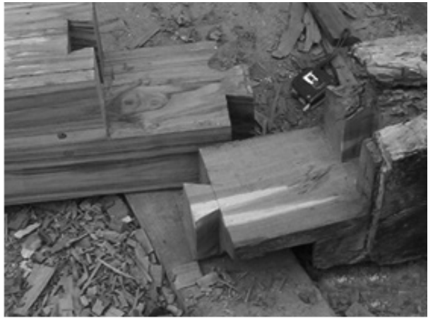
MS steel capping at joist end to reuse bulk of the original timber
