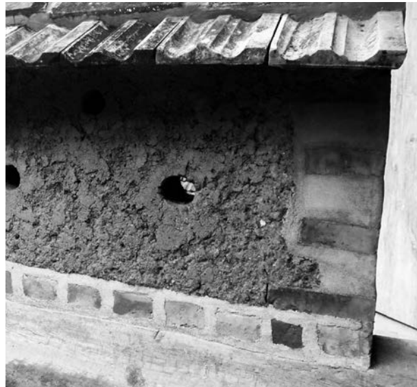
Terrace parapet. Source: Prakhar Tandon
