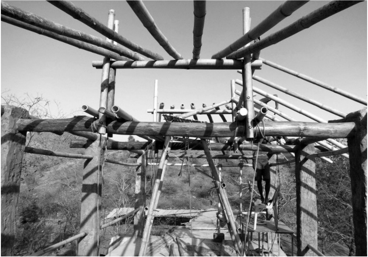
Basic roof structure using eucalyptus logs under construction
