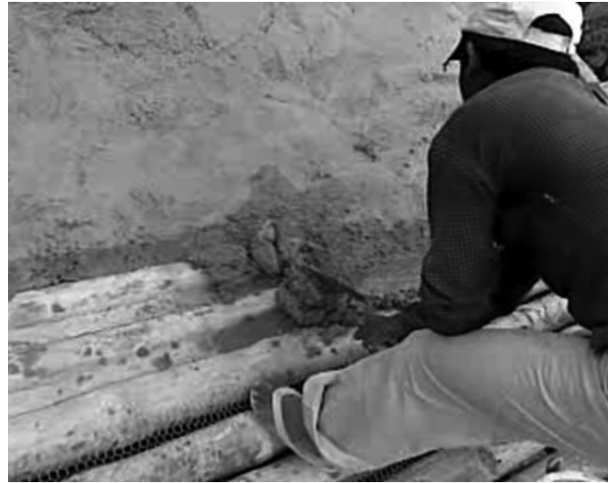
Mud over bamboo floor. Source: Prakhar Tandon
