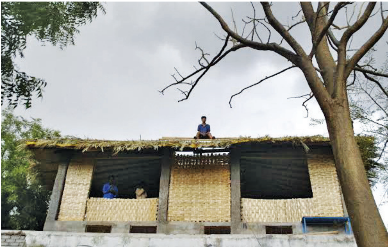
Woven bamboo mesh as wall over bamboo support structures
