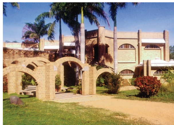
A series of welcoming CSEB arches guiding tourists into the Auroville Visitors' Centre
