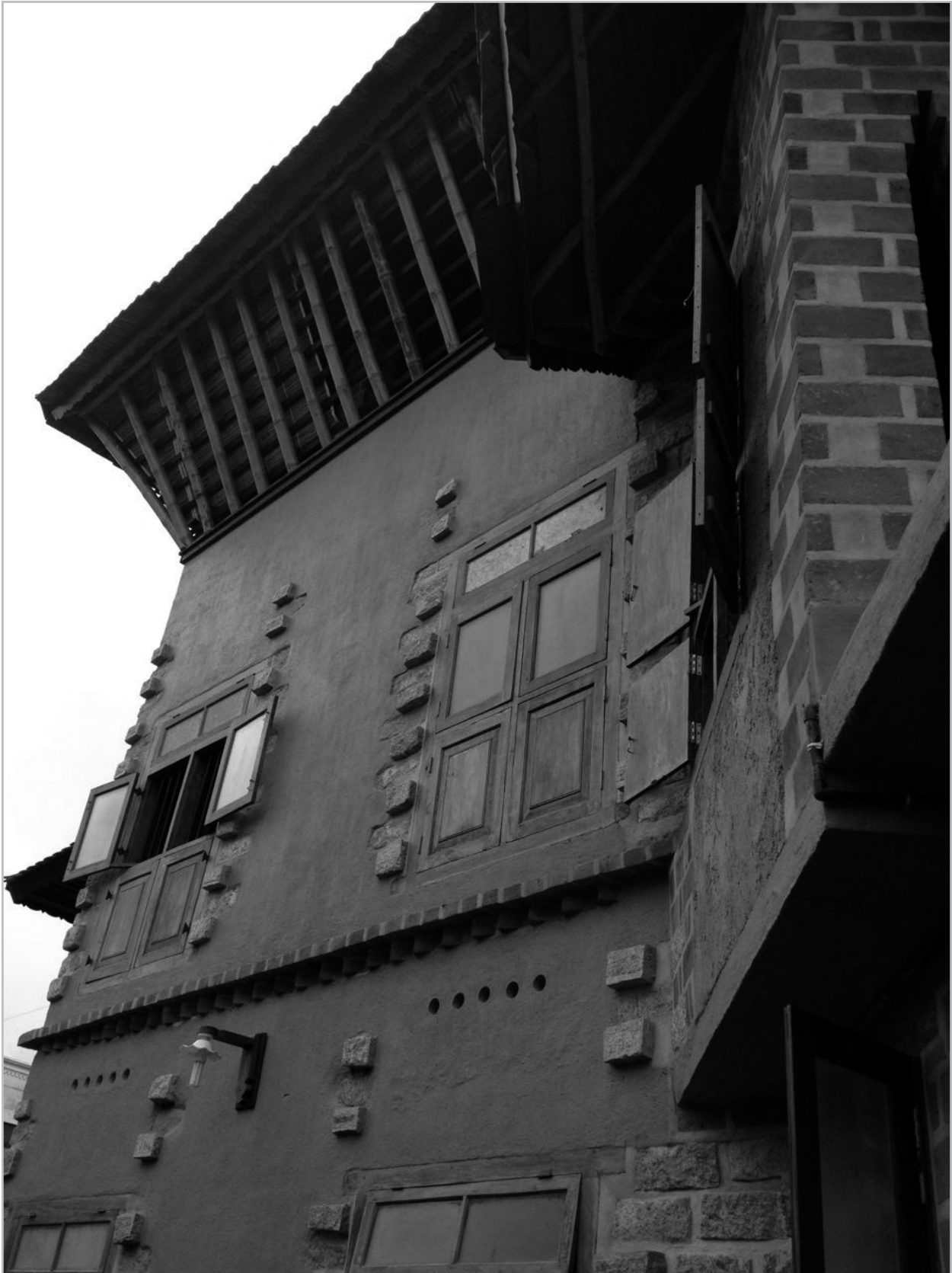
Water repellent paint finish
