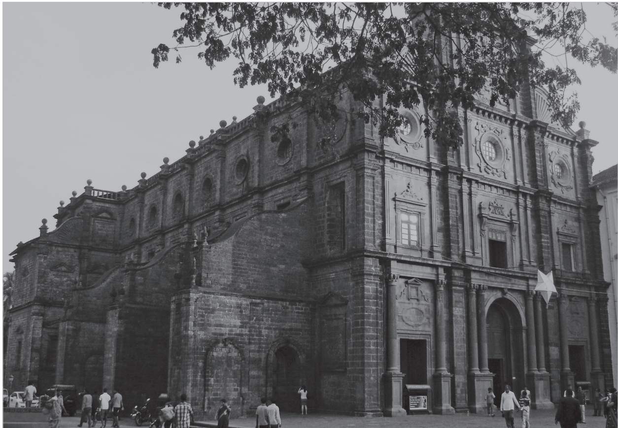
The towering Basilica of Bom Jesus in Goa constructed with laterite block
