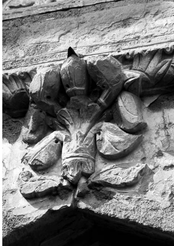
Lime stucco work, Bilhari
