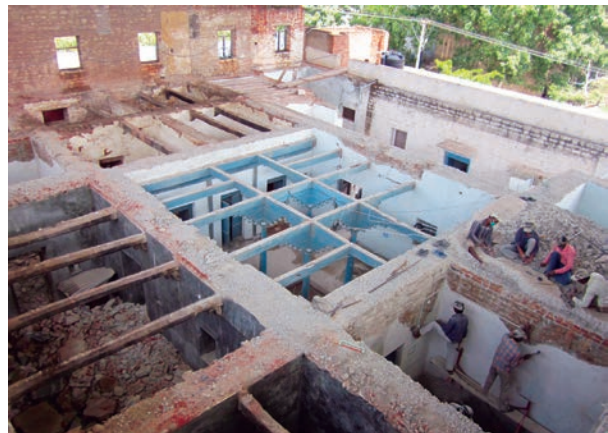
After removal of decayed timber. Source: RGRA project in Aneondi, Karnataka
