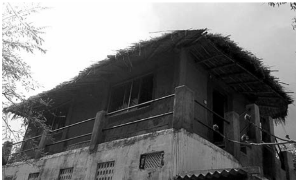
Mud plastered over woven bamboo mesh acting as walls
