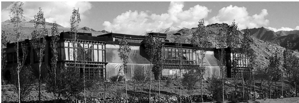
SECMOL's glass and rammed earth walls soaking in the mountain sun near Leh
