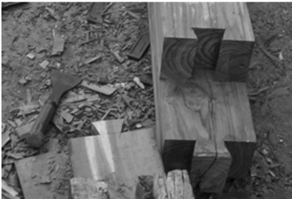
Restoring the roof structure of Ahilya Wada, Maheshwar, RGRA, 2005 with old and new timber using variety of joinery techniques
