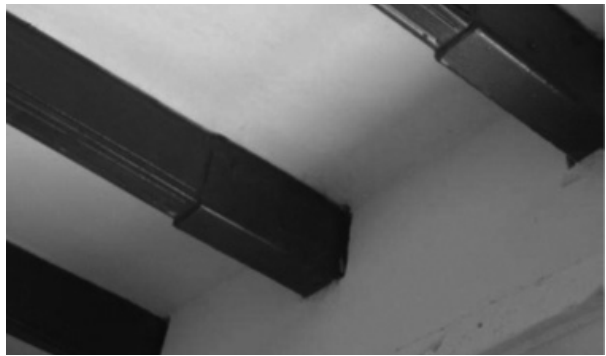
MS steel capping at joist end to reuse bulk of the original timber
