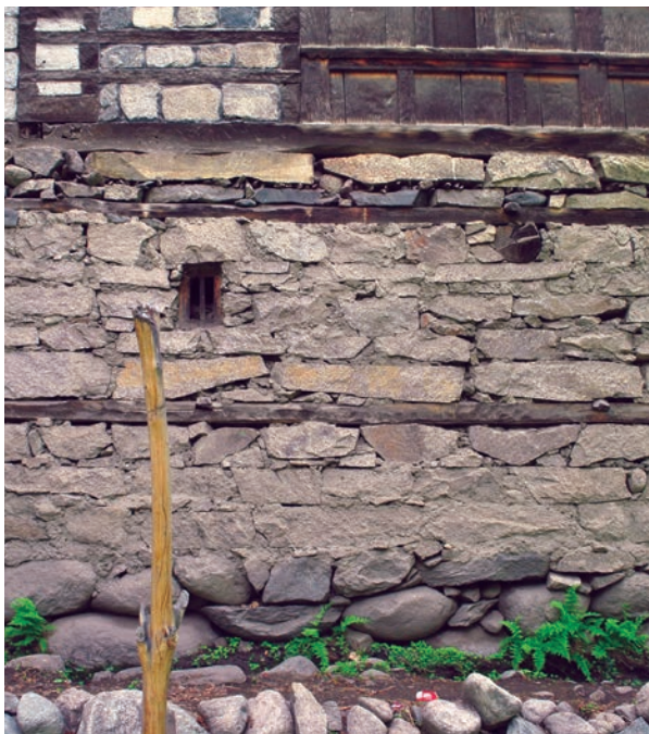
Typical stone masonry in Ladakh
