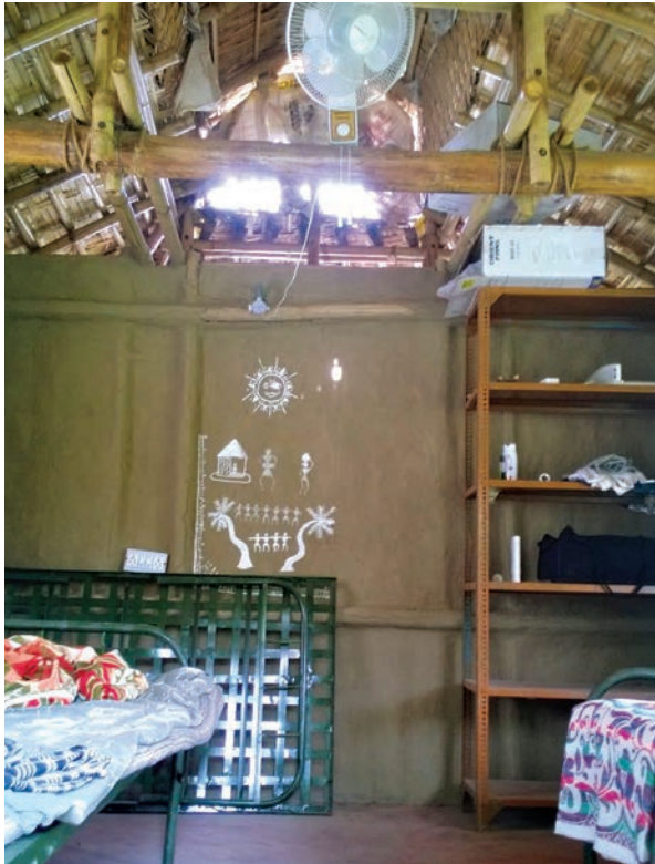
Interior spaces of the structure
