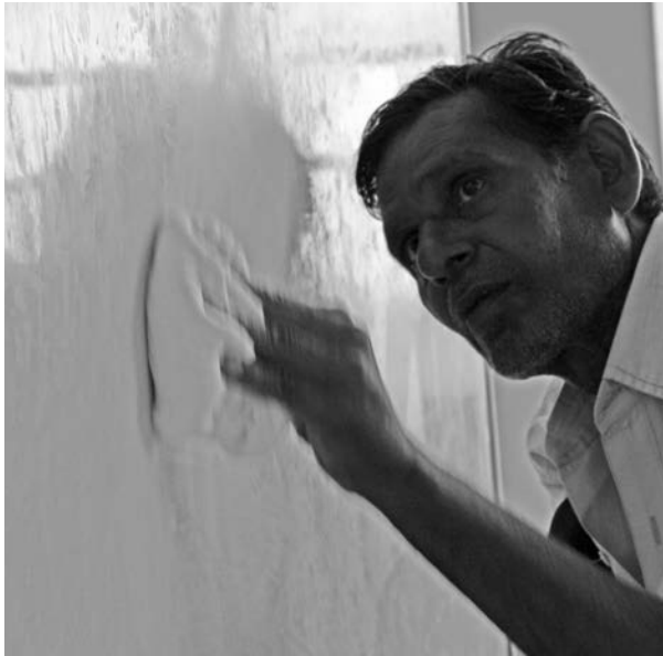
Finishing the final Araish layer
